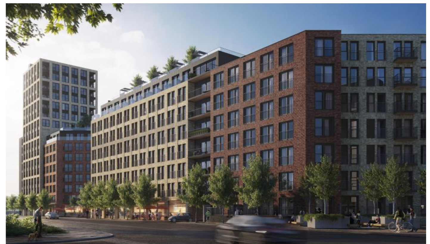
20/01543/MJR: Apartments, Anchor Court, Dumballs Road (Under Construction)
