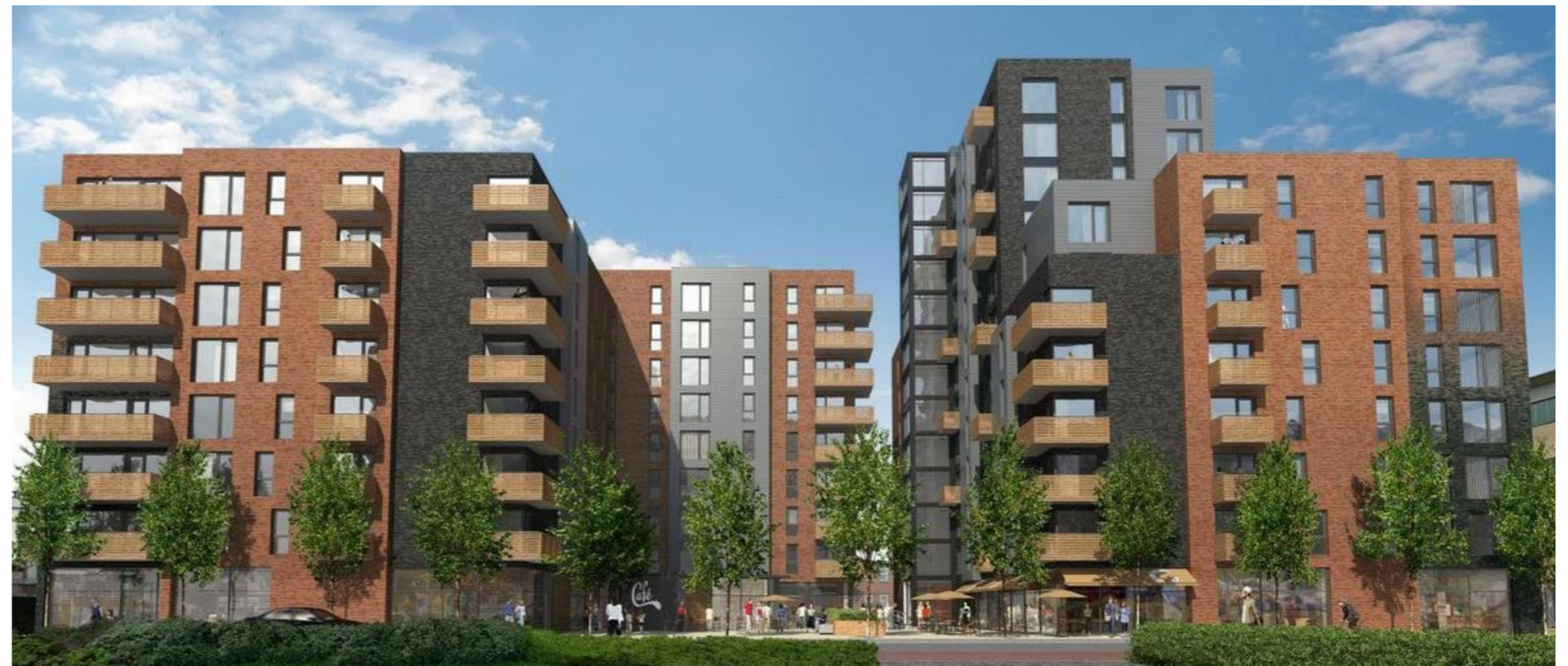
17/02404/MJR: Apartments, Dumballs Road (Under Construction)
