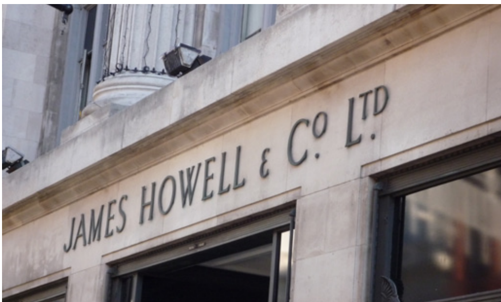
Figure.13 Lettering attached to stone
