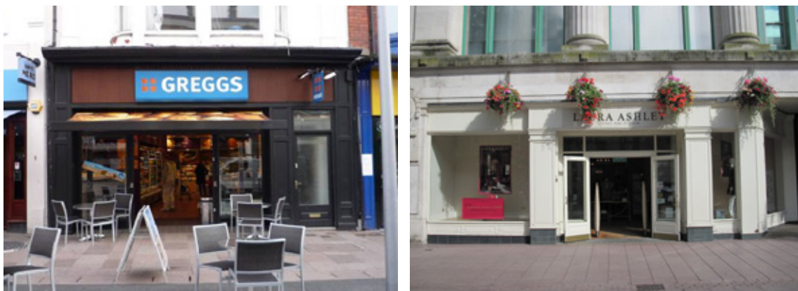
Figure. 19 Modern shop front altered to allow for a wider entrance
