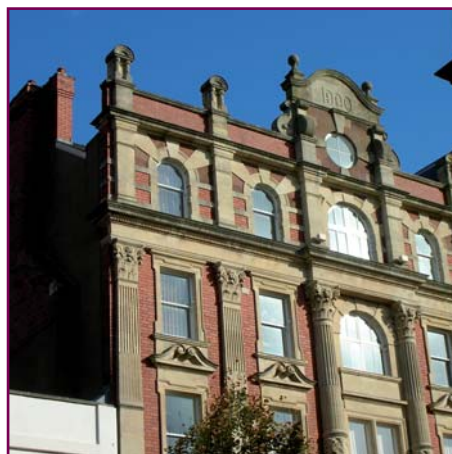
A mix of window styles including round headed windows with radial keystones, a round attic window and square headed windows with scrolled pediments.
