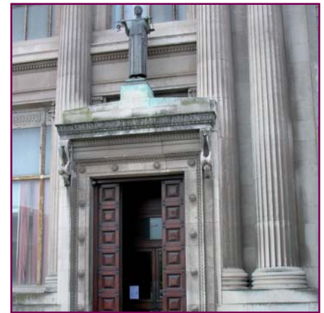
A statue of Equity stands on the cornice above the imposing doorway of the National Westminster Bank. The ground and first floor are framed by giant order fluted columns.
