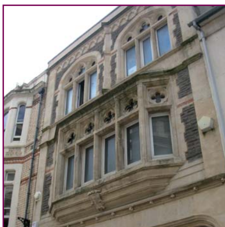
A former domestic building in Bute Street has been re-fronted in a Gothic revival style. Architectural features include an oriel window, stone tracery and small, inset roundel windows.
