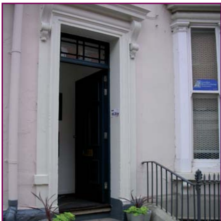
The wood panel door and fanlight on the former house is framed by a classically detailed doorcase with a simple hood resting on scrolled brackets.
