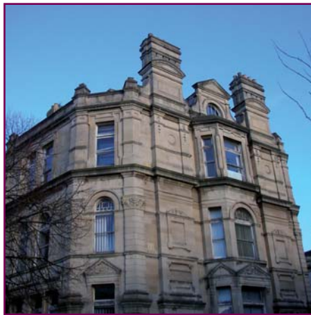
Prominent chimneys on the Cardiff Coal Exchange.
