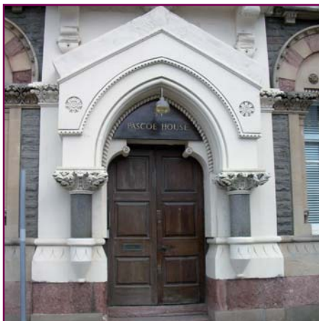
Impressive door surround displaying gothic influences. It includes a decorative hood resting on engaged granite columns which are topped by ornate capitals.
