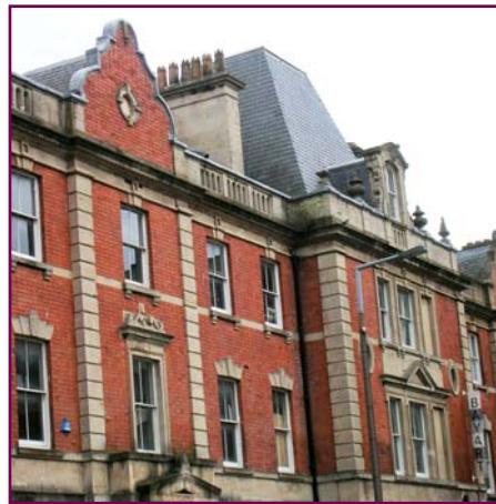
Dutch gables, chimneys and the roof form create visual interest at roof level.
