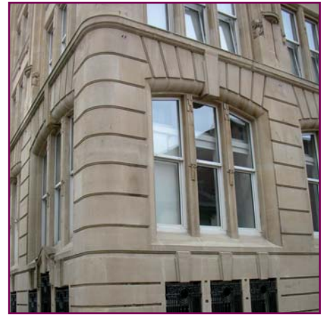
Rusticated stonework on the Cambrian Building emphasises the solidity of the building adding to its powerful appearance.
