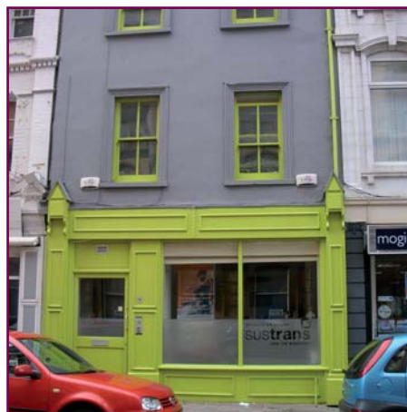
A shop front refurbished in a traditional style. It features a low stall riser, a timber mullion dividing the window pane, pilasters and console brackets.
