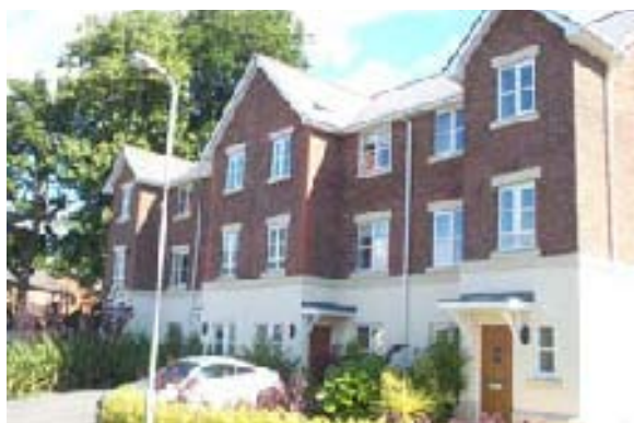
Fig.5 Maes Yr Anedd: New housing that employs a traditional vernacular and features quality materials and design features, such as the projecting eaves, window detailing and varying ridge tiles.
