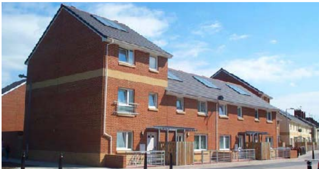
Fig.64 Recent developments at Allerton Street and Angelina Street feature integrated solar hot water systems.
