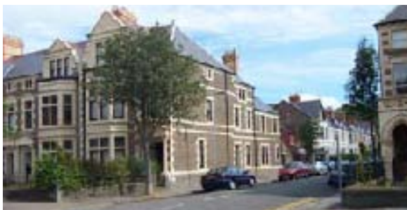
Fig.10 Cathedral Road - Building height used to differentiate between primary and secondary streets.
