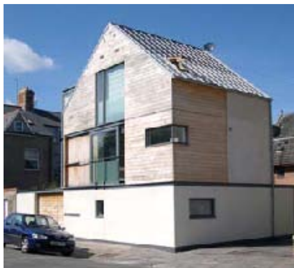
Fig.65 The Coach House – Constructed with recycled materials and sustainably-sourced timber and insulation (Thermafleece).
