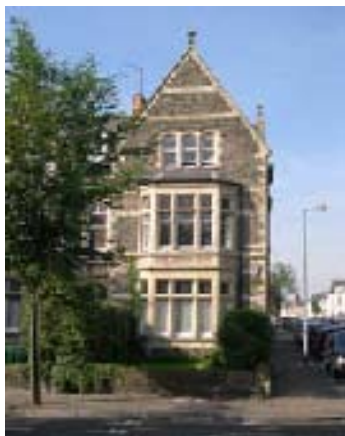
Fig.13 Ninian Road – Ends of terraces punctuated by gables.
