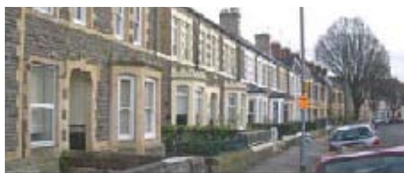
Fig.38 A typical street. A tight terraced form maximising continuity, enclosure and overlooking.
