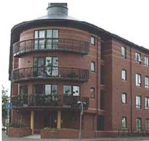
Fig.54 This building frames the junction, features active rooms on the outward facing elevations and has good sightlines over the streetscape.
