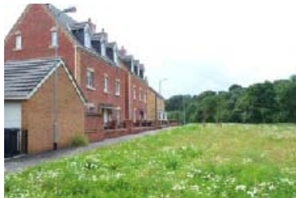
Fig.59 Radyr Sidings – This development has been designed to respond well to the adjacent Radyr Woods community nature area, which features a local nature reserve.
