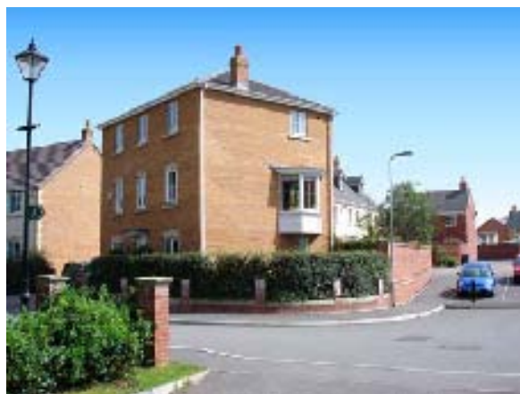
Fig.56 Junction Terrace, Radyr Sidings: This house turns the corner and has a full view of the public realm, creating defensible space.
