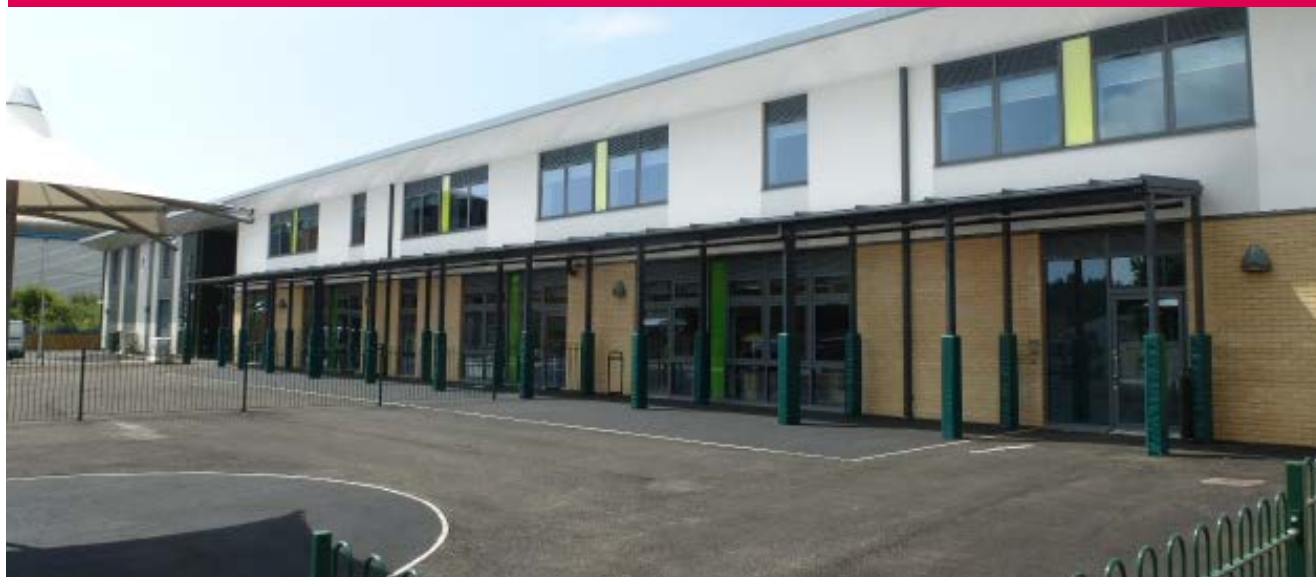
Recent new build primary school in Cardiff - Ysgol Glan Morfa
