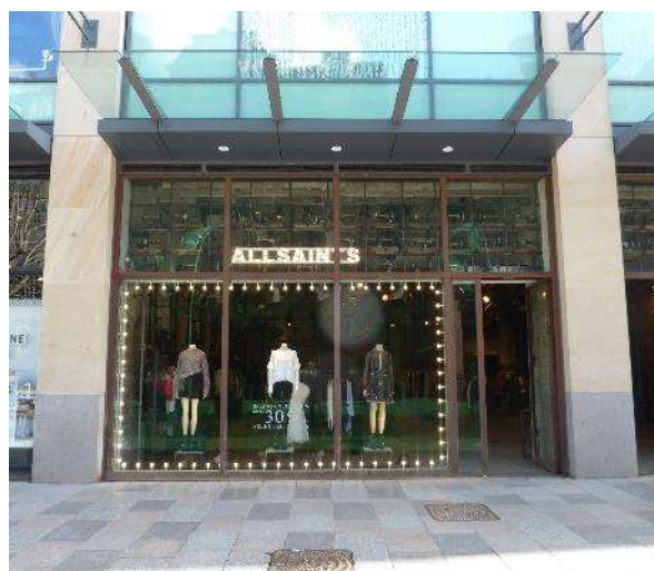
St David's Dewi Sant – Consistent shopfront proportions along The Hayes, framed by pilasters and glazed canopies
