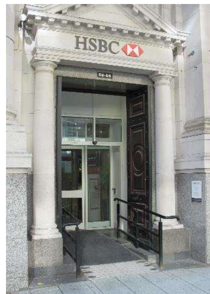
Listed Building ramp conversion
