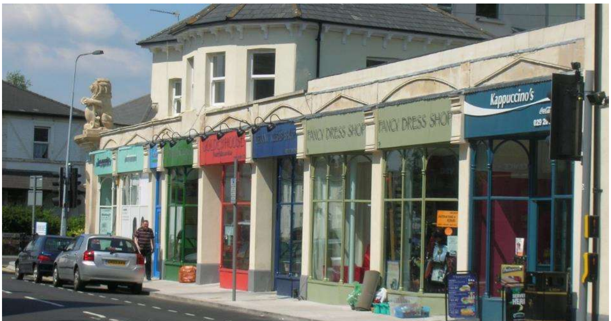
Consistent application of fascias and stallrisers across a group frontage - Clifton Street
