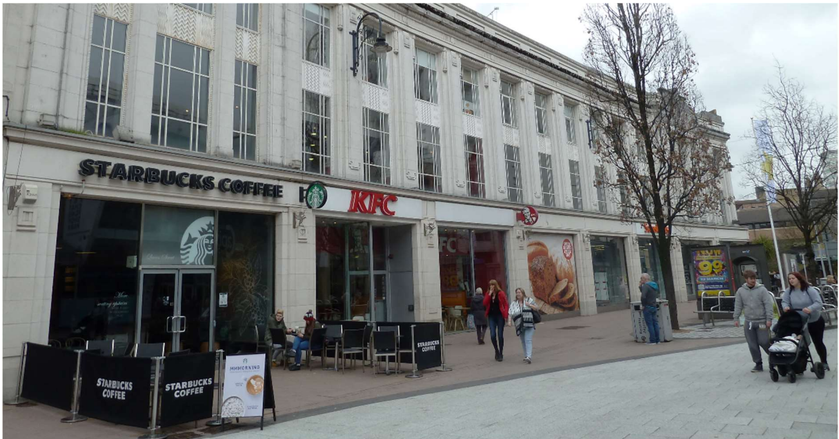
Consistency of bay widths and positioning of pilasters across a group frontage - Queen Street
